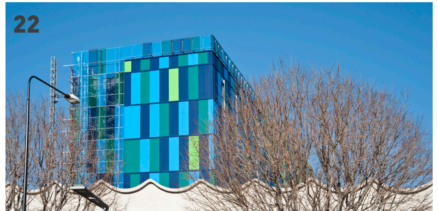
Vertically installed Trimoterm FTV facade system includes prefabricated L-shaped corners.
